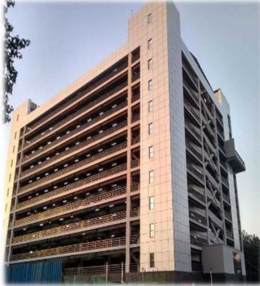
Sir Ganga Ram Hospital – Multi Level Car Park, Delhi
