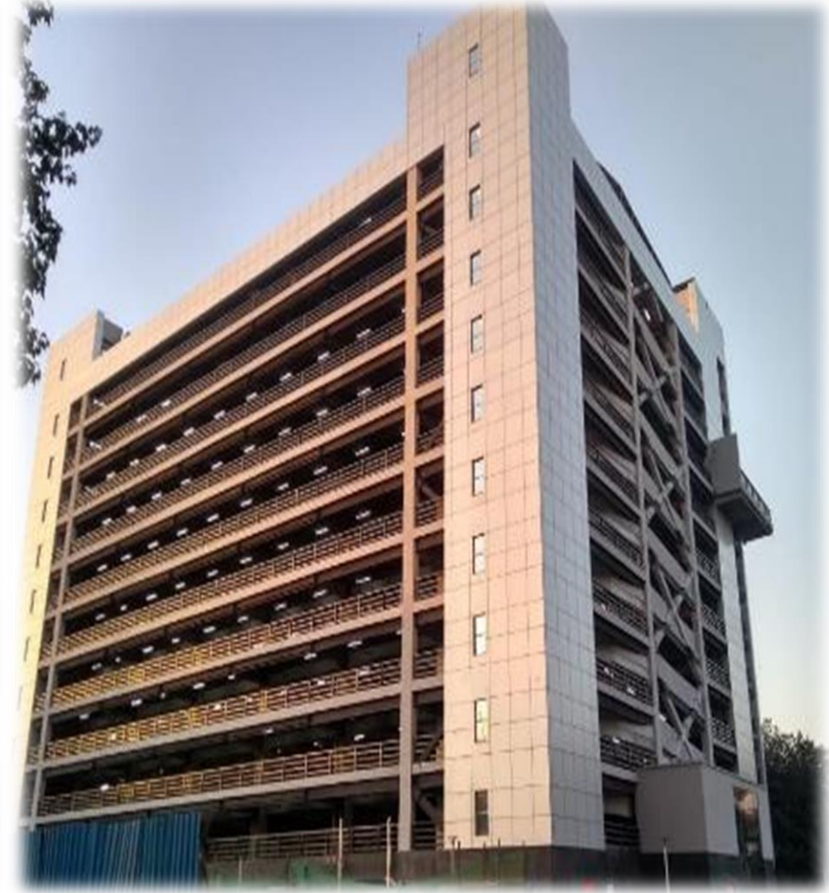
Sir Ganga Ram Hospital – Multi Level Car Park, Delhi
