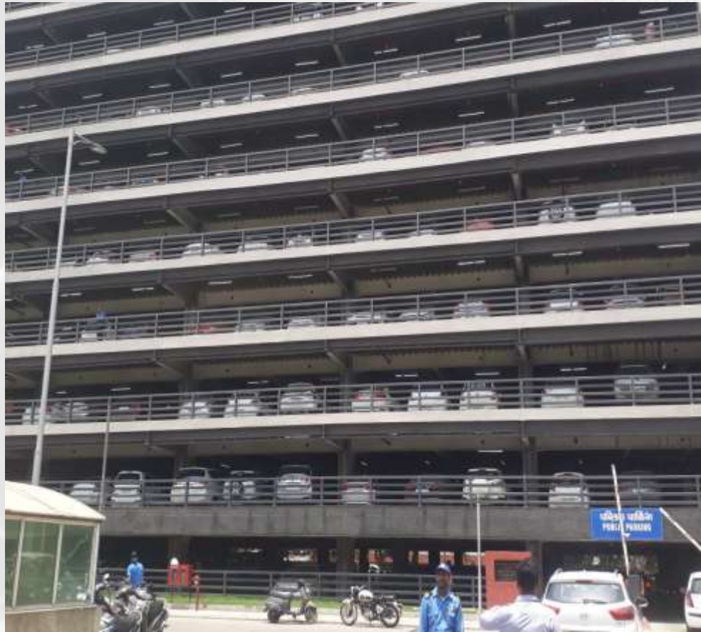
Sir Gangaram Hospital, Multi level Car Parking, Delhi
