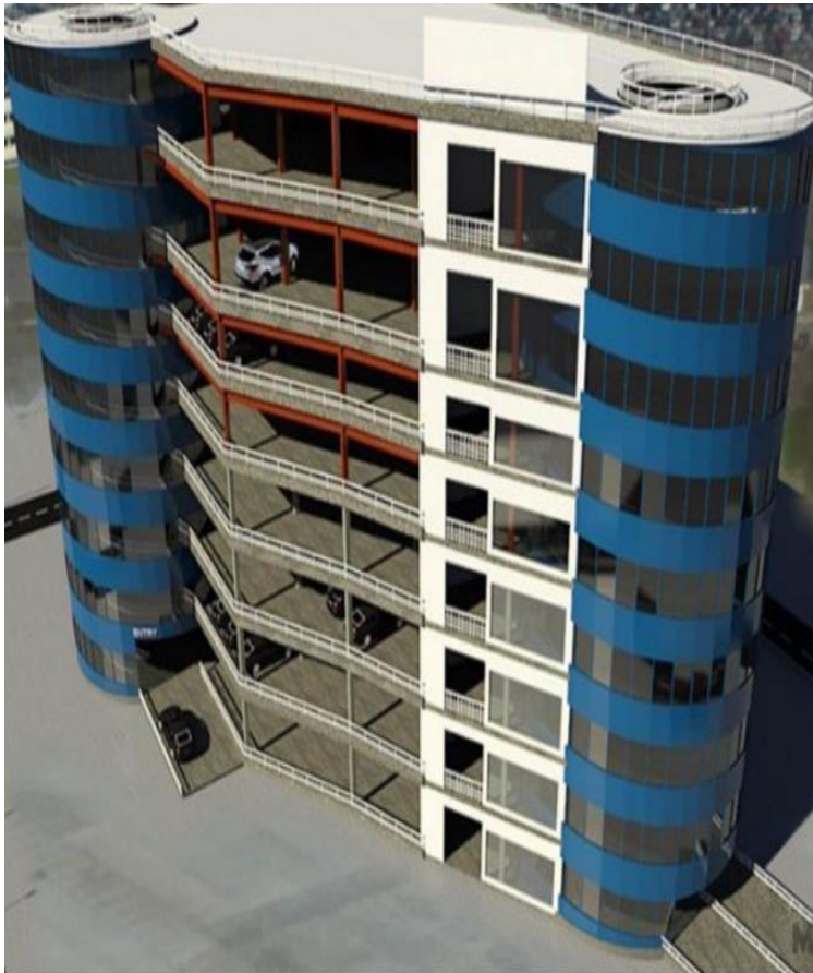
Sir Gangaram Hospital, Multi level Car Parking, Delhi
